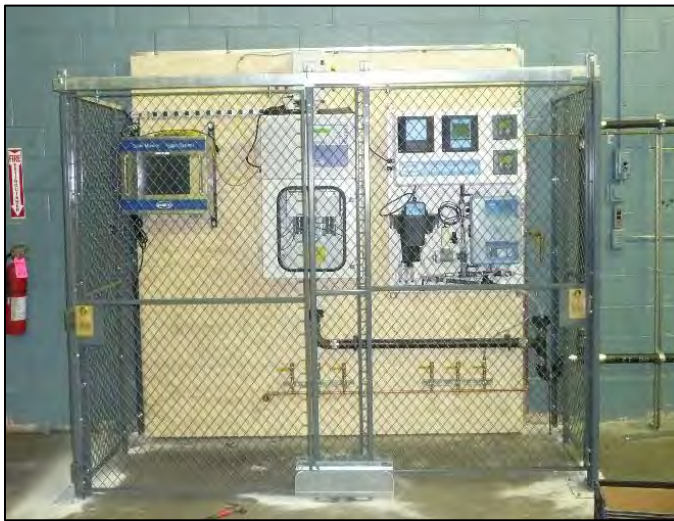
Figure 2-2. Wall-Mounted Rack with Protective Cage
