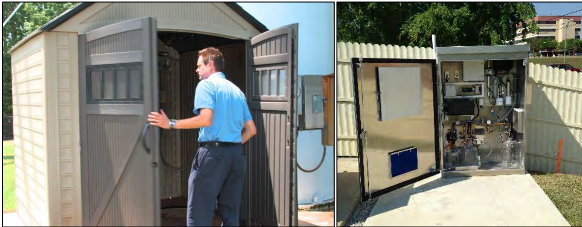
Figure 2-4. Enclosed Station Installations (Prefabricated and NEMA Enclosures)
