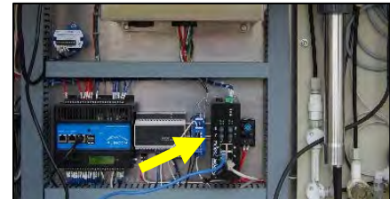
Figure 3-9. Ethernet Switch
