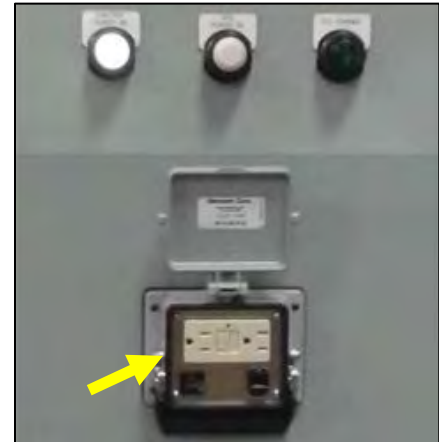
Figure 3-8. Panel Interface Connector
